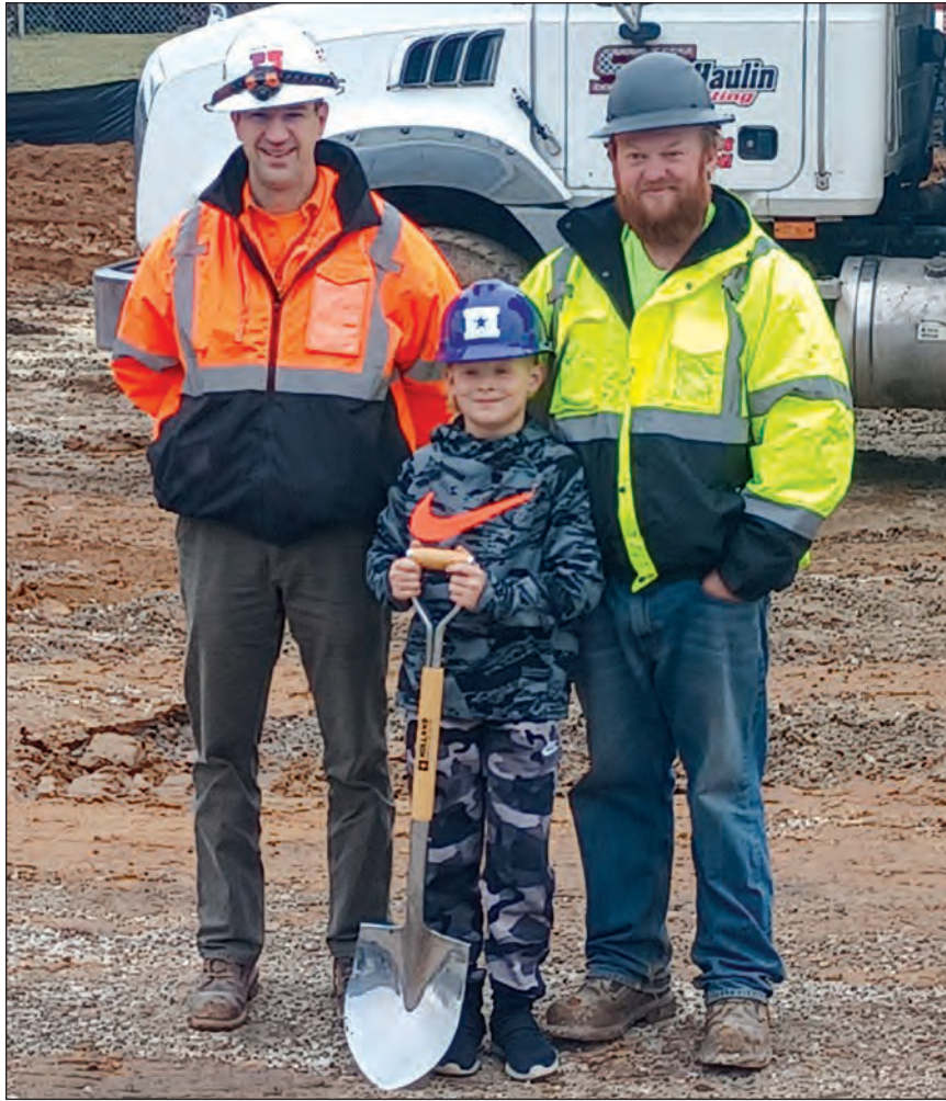
Holland Construction Superintendent James Bearden poses alongside Sammy Shafer of Shafer Excavating and his son Seth, a 4th grader at Caseyville Elementary School, as they stand at the site of the new elementary school. Photos by Devese "Dee" Ursery
